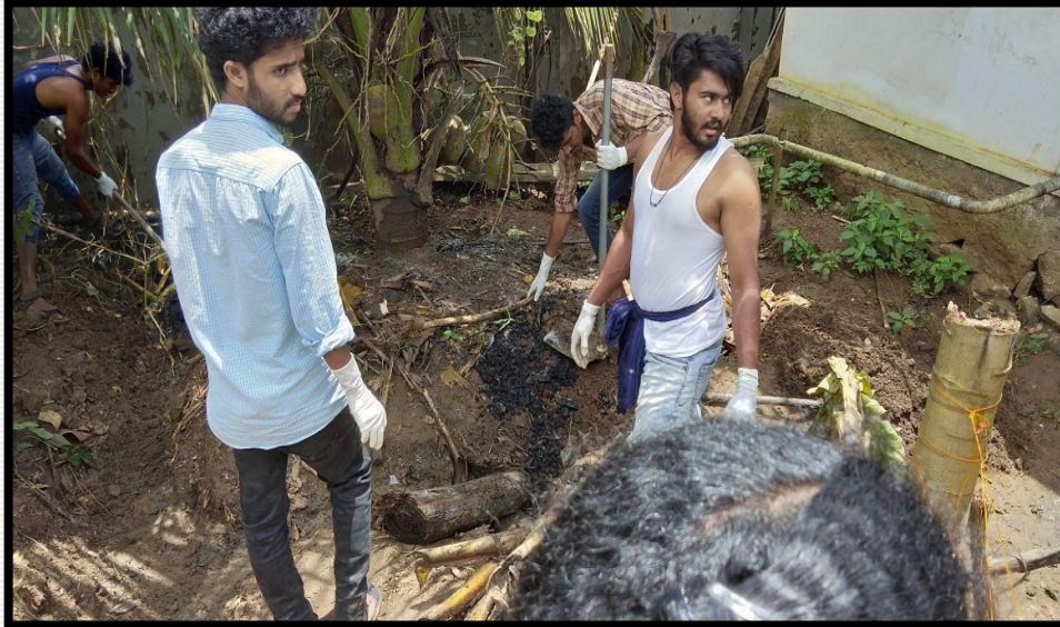
Cleaning Chekadi school site after flood relief camp
